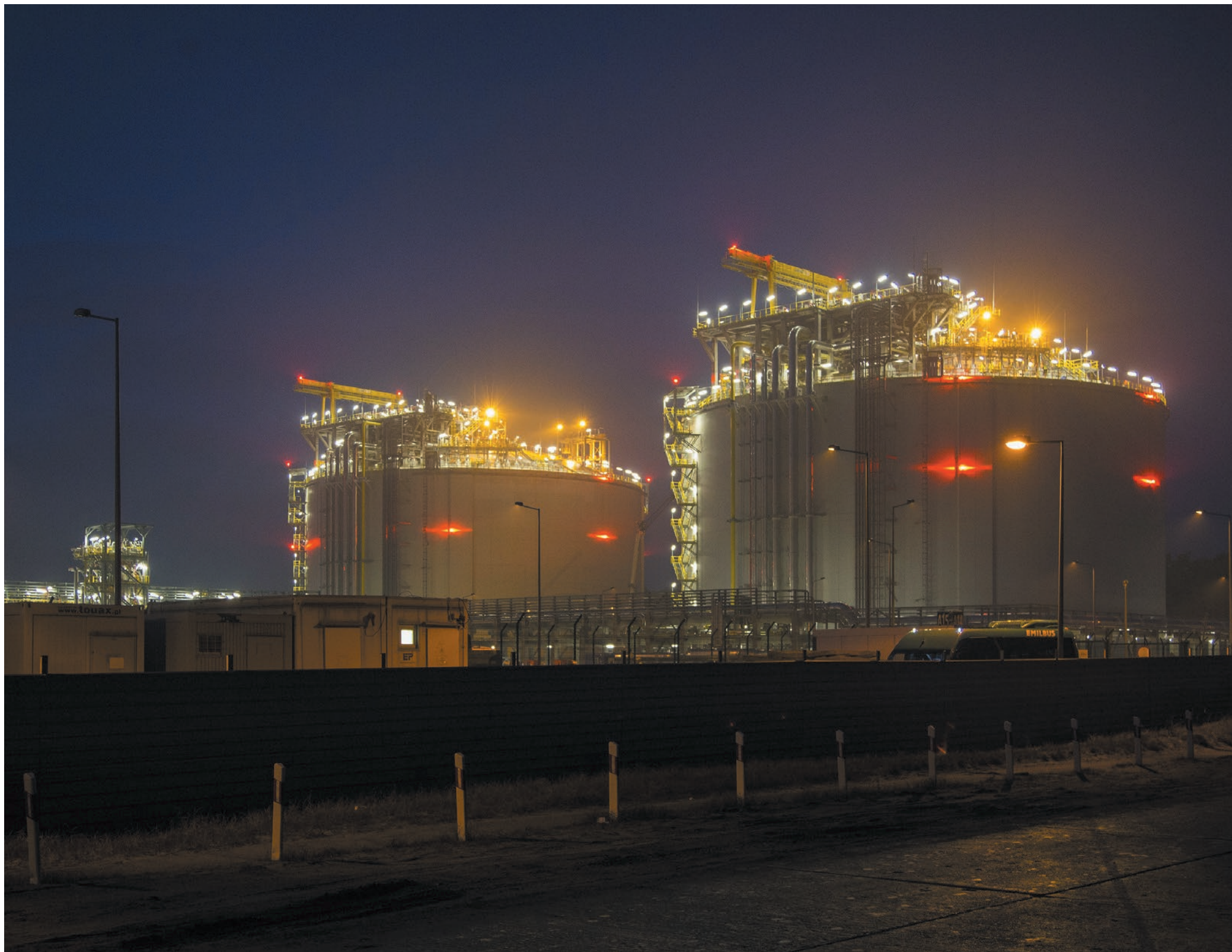
LNG terminal in Świnoujście (Baltic Sea) during the last days of its construction on 8 December 2015.
